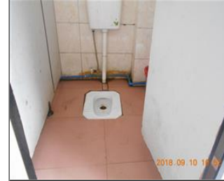
Photo of the sanitary facilities Toilet.jpg
